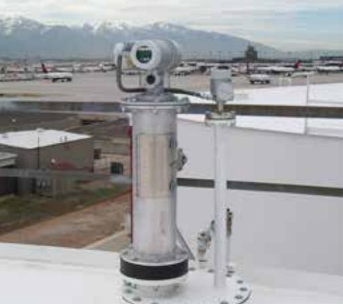
► In addition to level measurement with an accuracy of +/- 0.7 mm, the 6005 STG provides complete measurement of jet fuel, including interface level measurements of up to three liquids, density and tank bottom. In conjunction with the 4532 ATC, the 6005 STG provides complete and accurate fuel measurements throughout the tank.
