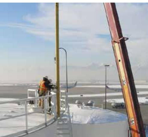
► The 6005 STG's high accuracy and multi-measurement capabilities are ideally suited for jet fuel applications. In order to take advantage of the high accuracy multi-measurement capability and operate to API standards, a fiberglass stilling well was fitted to each tank.
