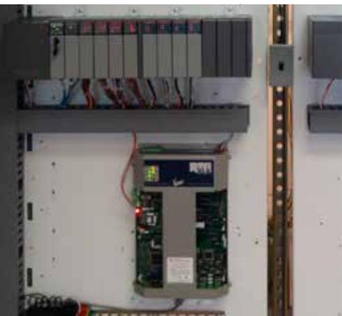
► Varec's 8130 Remote Terminal Unit provides system connectivity to the servo tank gauging system and expandable functionality for future facility automation and integration.
